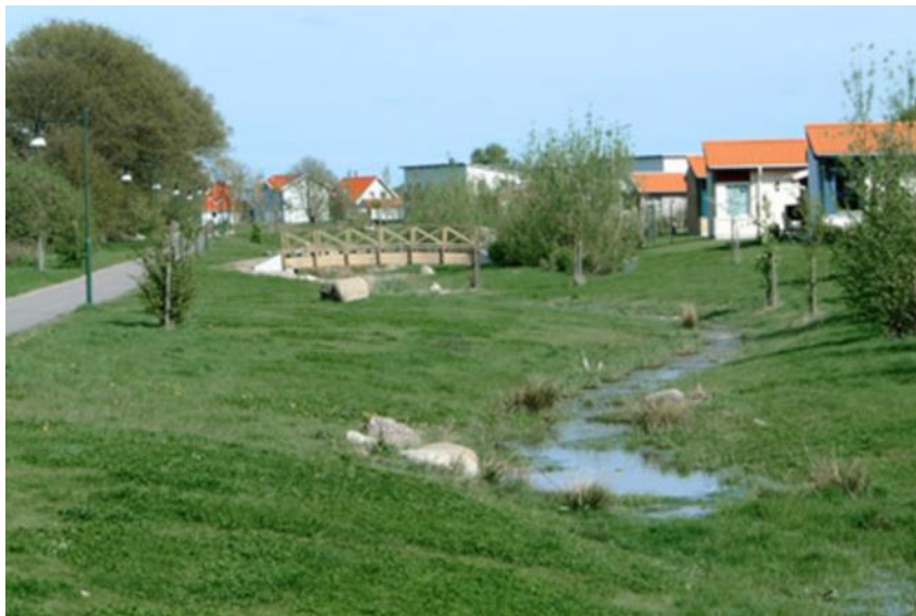
Figur 3.2.2 – utformning meandrande diken, princip (foto NSVA)
